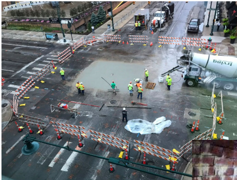
Initial Intersection Closure and Saw-Cutting of Street Prior to Excavation to Maintain Asphalt Integrity
