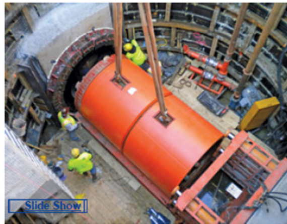
Photo: Courtesy of Indianapolis Dept. Of Public Works Tunnel boring machine in the Belmont North Relief Interceptor, added to the plan.
